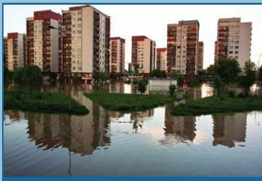
Flooded streets in Wrocław, Poland (June 2010) [1]
